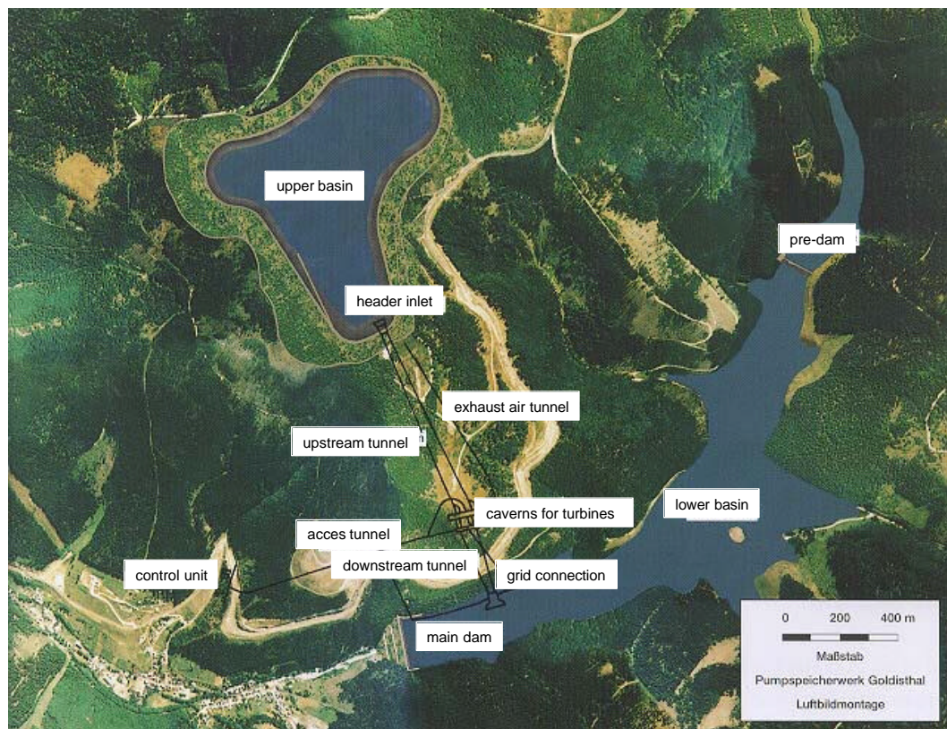
Figure 1-10: Pumped hydro power plant Goldisthal (Walter Bau AG)
